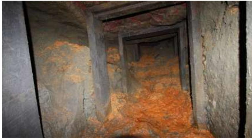
Figure 7: Vertical soil between 2 wooden frames in an unfinished tunnel of the Zonnebeke Dugout (photo Ingenieursbureau Norbert Provoost bvba)
