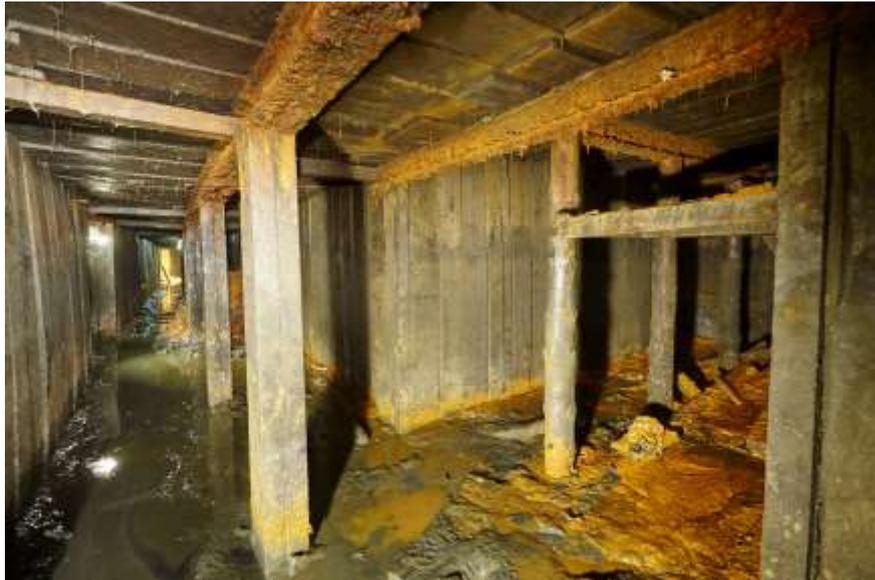
Figure 3: Central tunnel and adjacent room equipped with the remains of racks used as bedding for military in the Zonnebeke Church Dugout, 100 years after its construction by Canadian and Australian Tunneling Companies (photo K. Vandevorst - Flanders Heritage Agency)
